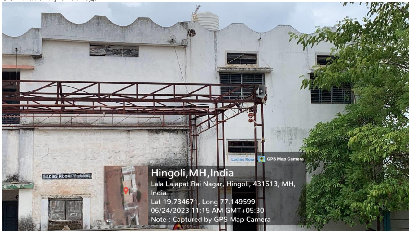
CCTV near Girls Common room
